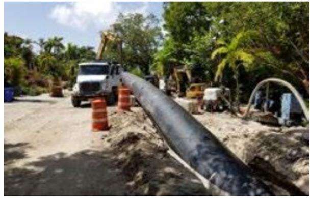
Construction of a new 7.5-mile redundant forced main sewer required two contractors using horizontal directional drilling (HDD) to install the 54-inch diameter HDPE pipe. Murphy Pipeline Contractors, Inc. (Jacksonville, FL) ran from the north while David Mancini and Sons (Pompano Beach, FL) came from the south. Both companies are contractor members of the Municipal Advisory Board, an independent, non-commercial adviser to the Municipal & Industrial Division of the PPI.
